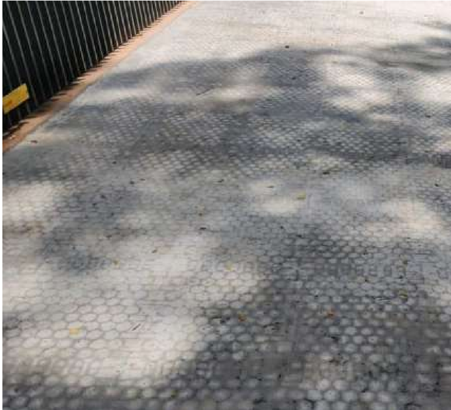
Entrance Ramp at ABB Factory with GridMats
