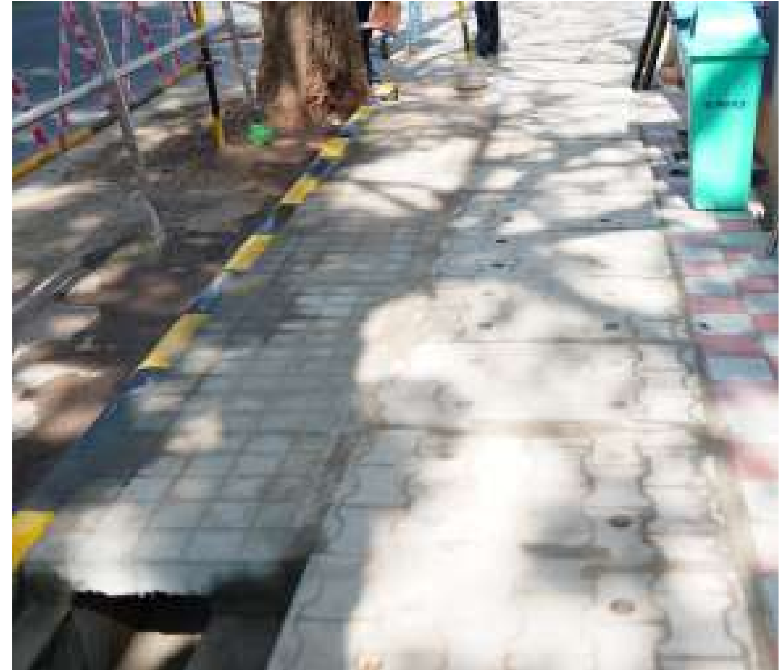
2KMS of drain cover slab reinforced with GridMats
