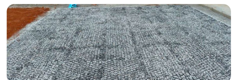
Brushed flush with the cell tops
