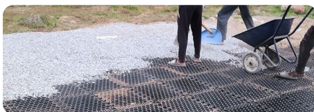
Chips filled and compacted flush
