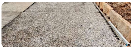
Kerbed access road, opened the same afternoon
