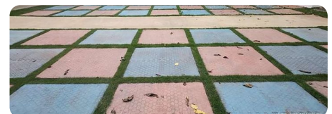
Pavers before the grass closes over
