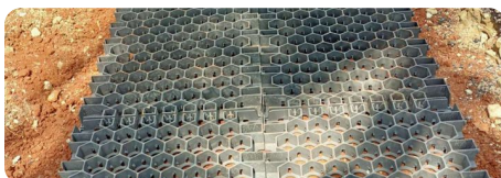
Laying OC-LW for a soil finish
