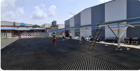
1 Grid laid on the compacted base: RINAC, Mumbai, on OC-LW 40
