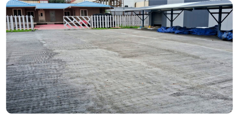
3 Finished truck yard, moist-cured 3 days: RINAC, Mumbai, on OC-LW 40
