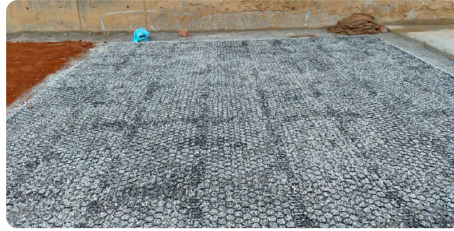
2 Filled with cement-treated chips, compacted and brushed flush
