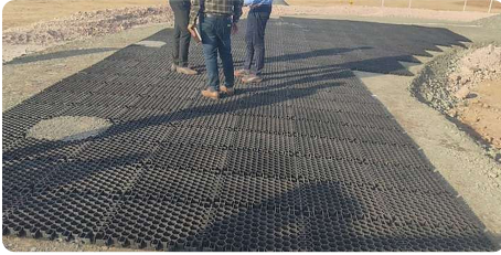
1 Grid laid and clipped on the compacted base
