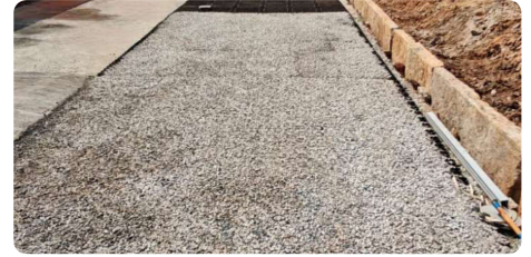
3 Plate-compacted, kerbed and open the same day
