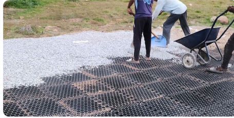
2 Clean angular chips filled into the cells
