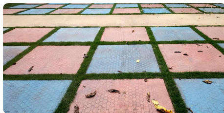
2 Root zone filled; the grass starts to close over
