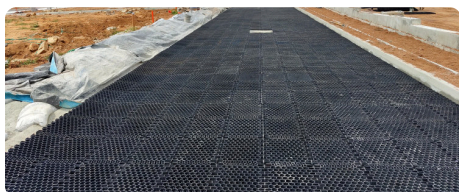
1 OC-HD 40 laid on the lean-concrete bed
