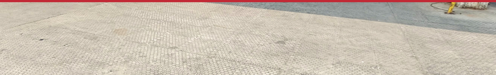
PGP Glass, Gujarat: honeycomb-finish apron at the loading bays; the cell tops are the finish
