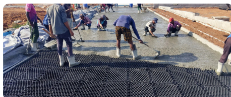
2 Concrete placed and finished flush with the cell tops
