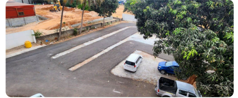
3 The finished road and parking: Orxa Energies
