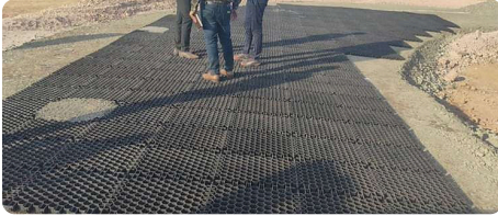
1 The grid laid in the granular base
