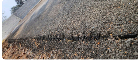
2 The asphalt goes on as before; the grid stays in the base
