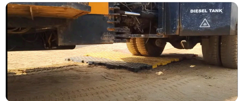
3 A loaded truck on the mats at a wind site
