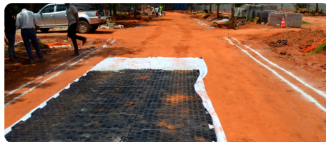
2 Laid as a temporary track over soft ground
